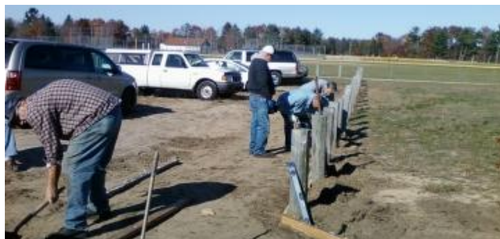
Lions preparing to pour cement at Mullally Park
